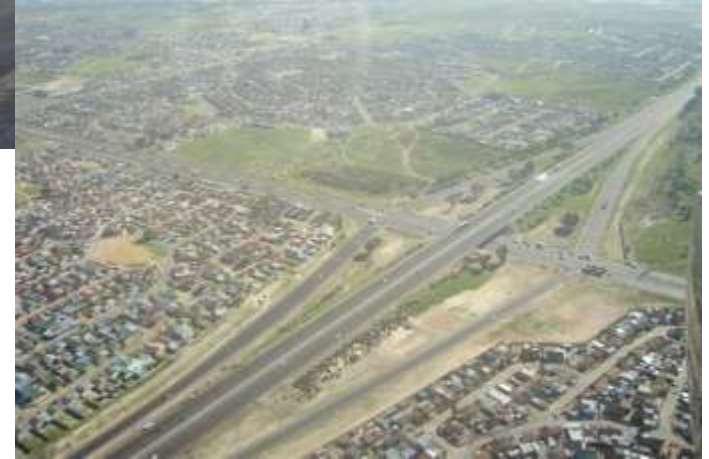
Cape Town – R300 Link Road R525 000 000
