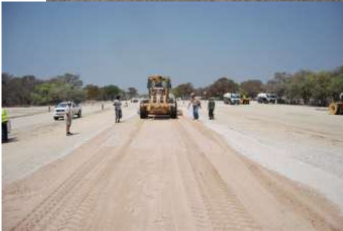
Namibia – Rundu to Elundu R1 001 000 000 To be completed Dec 2011
